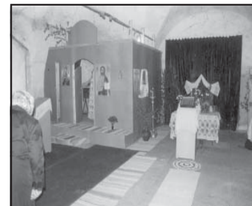
Interior Trapeza—Church of Archangel Michael under restoration
