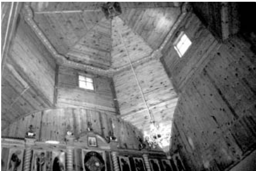
Interior of newly-roofed St. Nicholas Church.
