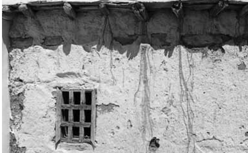
Ancient wall and window in the kitchen area before restoration.
