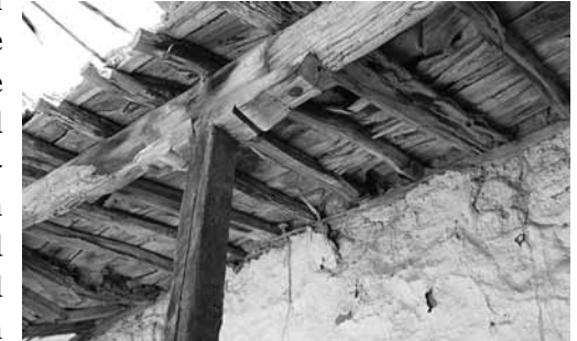
Use of branches and reeds in construction, from the scarcity of wood in the area.
